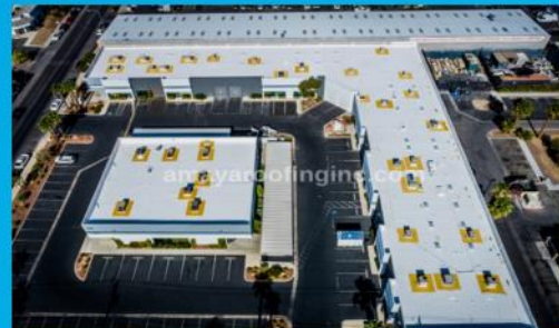
ROOF COATING RESTORATION
